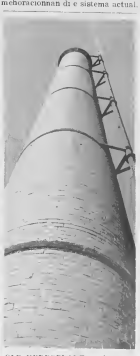
OLD HYDR-PLANT stack serves as flare support. Mechanically, the flares are relatively simple. CHINESE BIEUW of Hydro Plant ta sirbi como sostén pa e flar. Mecanicamente, e flar-cum ta relativamente simple den construcion.
